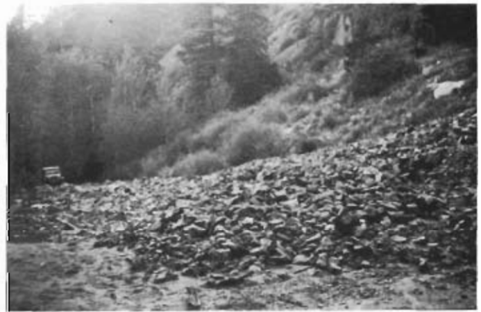
Figure 17.—Coarse rubble fan from the debris flow of September 8, 1980, buries the road to the USFS North Crestone Campground with up to 2 m of boulders. Intense local rainfall of 75 mm in 45 minutes triggered this event; evidence for older flows at the same location was noted.
