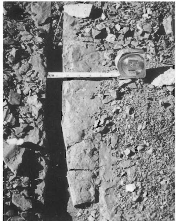
Figure 10. Photograph of open (dilated) joint on the floor of a 15-m deep cut into the State Bridge Formation (Permian–Triassic), approximately 400 m north of Loge Peak. Numbers on tape measure are inches. End of tape could be lowered 1.5 m into this joint.
