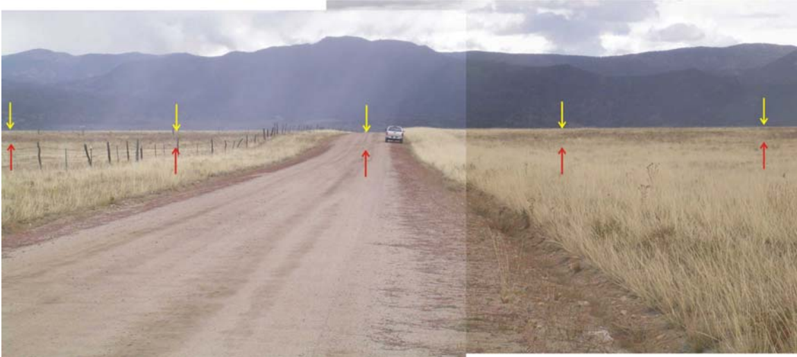
Figure 39. View of antithetic fault scarp (between arrows) offsetting Kansan alluvium (Qk) by 8.2-9.8 feet in Maxwell Park. View to east along County Road 328. Pickup truck on scarp is 7.2 feet high.
