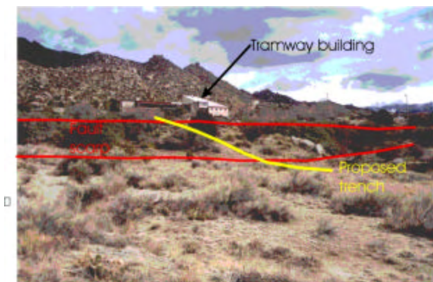
Fig. 9. Fault scarp of strand B of the SFZ (between red lines), south of Tramway Road. The Tram Station building is visible at center. Originally-proposed trench line is shown in yellow. Based on field reconnaissance, this part of the scarp was not disturbed during construction of the tramway parking lot (red circle on Fig. 4), which lies to the right of the Tram Station building.
