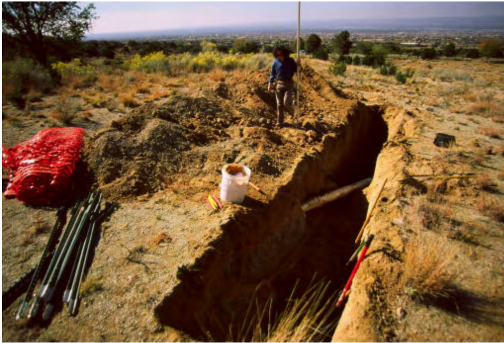
Fig. 11. Photograph of the initial trench, showing the NW-trending water line exposed in the trench. View is to the west.
