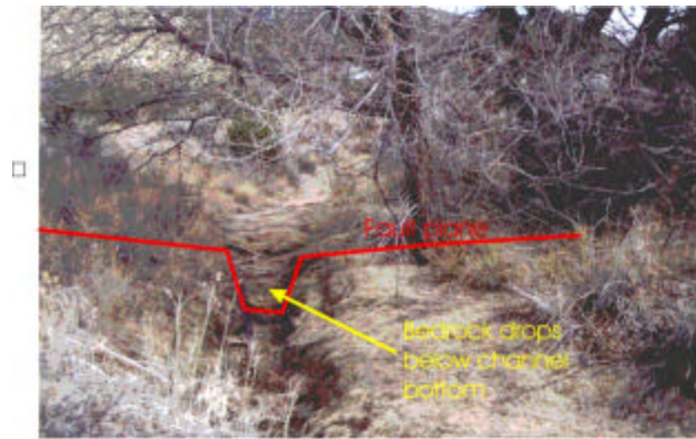
Fig. 6. Fault strand C of the SFZ (red line) where it crosses the gully north of the Tram Station. View looking east. East of the fault the gully flows on Sandia Granite, but bedrock drops below the gully bottom at the fault. Cottonwood trees at right are rooted in the fault plane, and form a lineament that crosses deposits of several ages, as mapped by Read et al. (2000). Photo by J.P. McCalpin, March 1, 2001.
