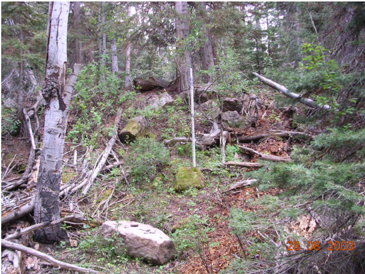
Fig. 21. The steepest, basal scarp in the Traver Mesa section; view is to south. Rod is 1.5 m long. Bedrock blocks behind the top of the rod dip 30^{\circ} N (toward the viewer) and slabs at mid-scarp position dip 50^{\circ} N.
