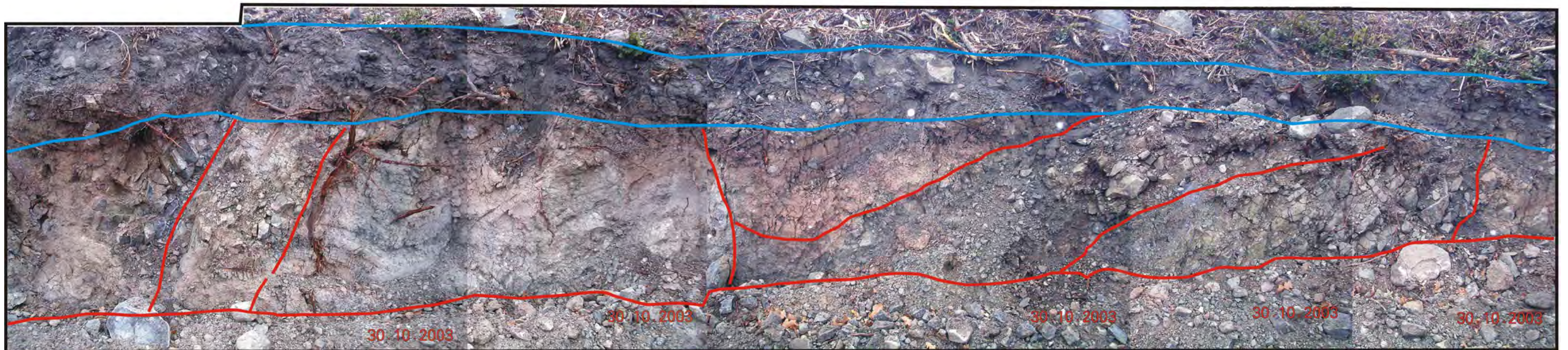
Fig. 4. Photo-mosaic of a south-facing roadcut on the southern margin of the 80-acre inholding in central Suncrest. Lower panel, annotated photomosaic; upper panel, interpretation.
