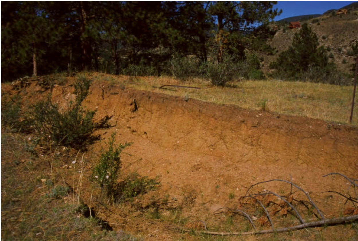
Fig. 5-13. Roadcut exposure of a soil profile at the crest of the Quarry Saddle, 59 m above stream level; view is to SW. Soil horizons and thicknesses are: A, 0-10 cm; B21t, 10-30 cm; B22t, 30-50 cm; B23t, 50-60 cm; B3, 60-90 cm; B4?, 90-130 cm; Cox, 130-160 cm.
